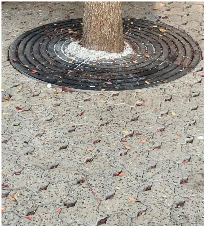
Permeable paving to surround existing / proposed street trees
