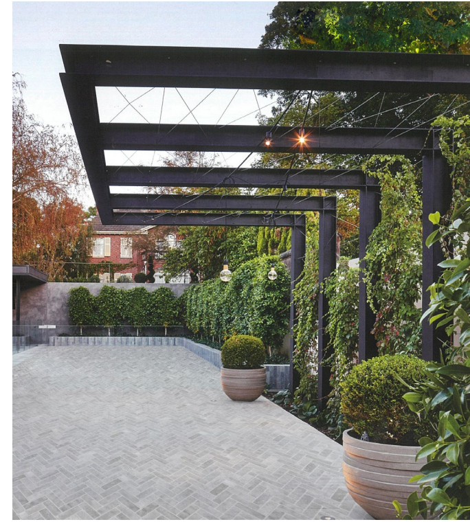
Steel framed arbour with climbing vine
