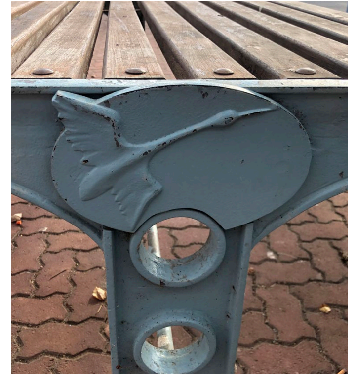
Existing picnic table (detail) - repaint, replace battens
