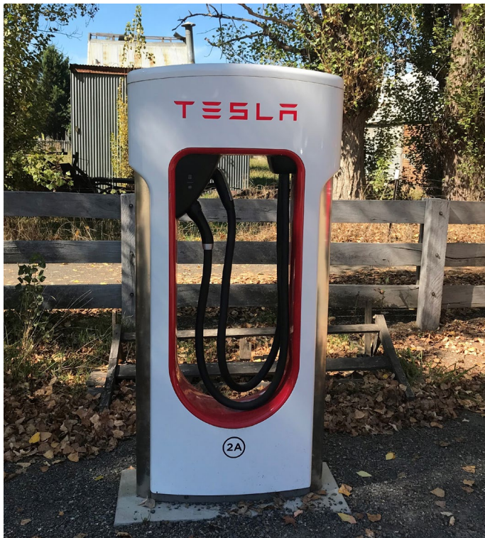
Electric vehicle charging station
