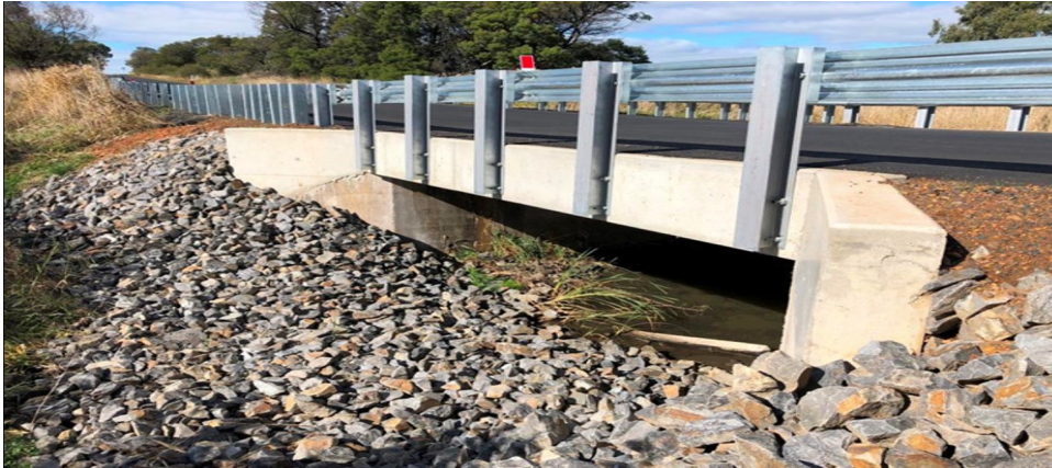
Kadnook Connewirricoo Road Bridge over Kadnook Creek – new deck overlay and guard rail
