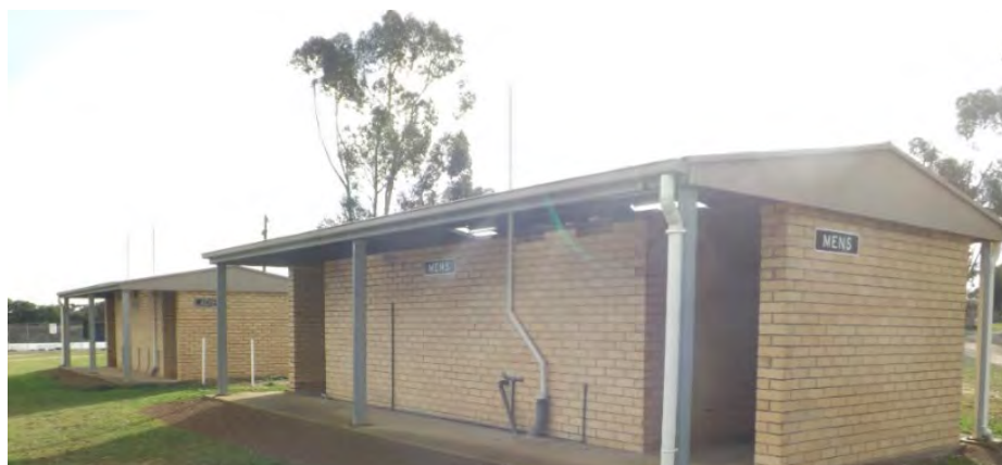
Figure 28: Upgraded sewer system works have been completed at the Kaniva Recreation Reserve Toilets.
