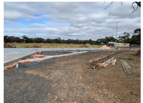
Figure 25: Goroke Recreation Reserve and Pavilion foundations have been laid.
