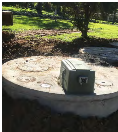
Figure 27: A new wastewater treatment system to be installed at Johnny Mullagh Caravan Park.
