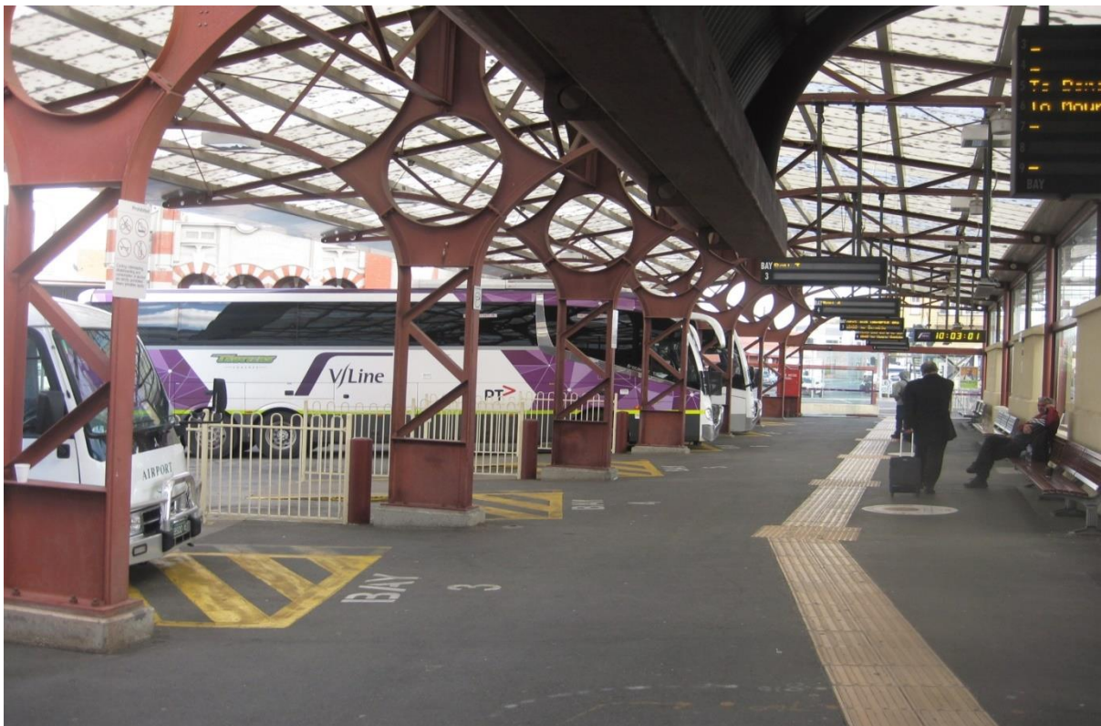
Figure 4: Road coach terminal at Ballarat Station
