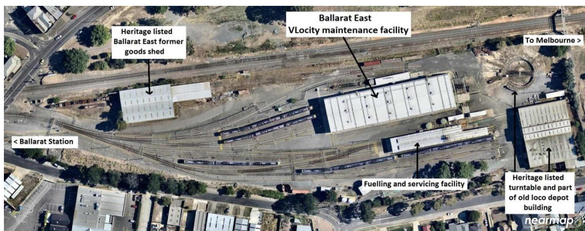
Figure 26: Ballarat East VLocity maintenance, servicing and train stabling facilities
