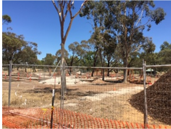
Construction begins on the new play space in Kaniva next to the Fauna Park
