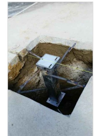
TYPICAL DETAIL FOR SLEEVE INSTALLATION - CUT OUT METHOD FOR CONCRETE PAVEMENT
