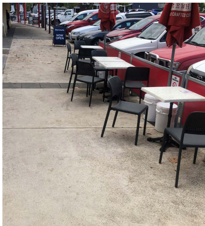
Standard concrete paving with tool joints in a grid pattern
