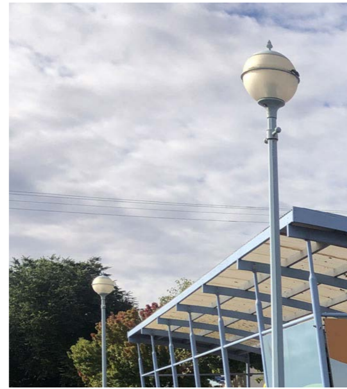
Existing lights - repaint
