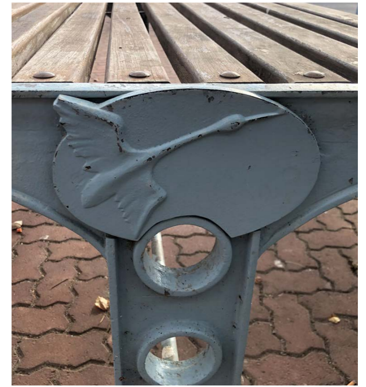
Existing picnic table (detail) - repaint, replace battens
