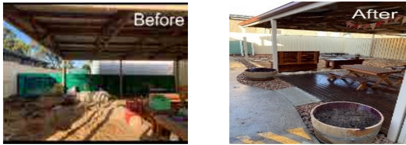
A collaborative approach between stakeholders enabled the Kaniva Kindergarten yard upgrade
