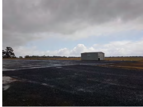
Facing north from hangar, across parking area to ambulance transfer building
