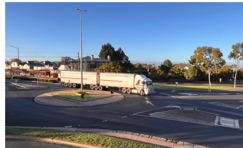
Roundabout, Commercial Street (E and W) and Madden Street (N and S), Kaniva
