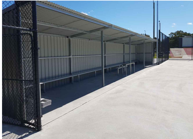
TYPICAL COLOURBOND DDA ACCESSIBLE 4.0(L) x 2.0(D)m LONG SCORER SHELTER AND 6.0(L) x 2.0(D) PLAYER SHELTER
