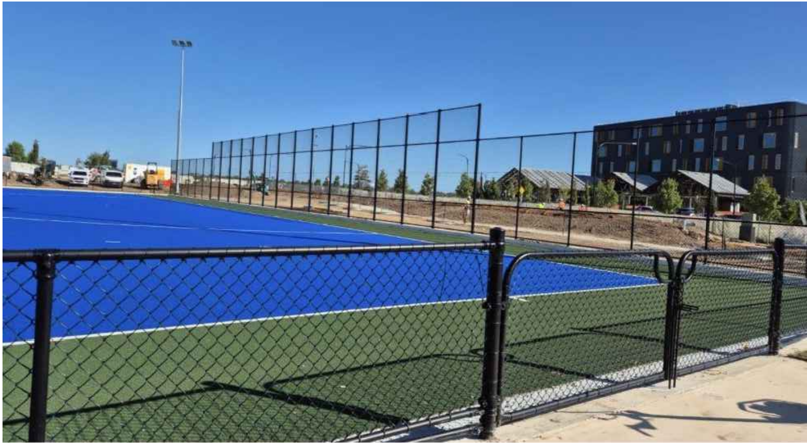
TYPICAL 6.0m HIGH FENCING BEHIND HOCKEY GOALS TO PREVENT AERIAL BALLS EXITING THE FACILITY AND INTO THE RESERVE.
