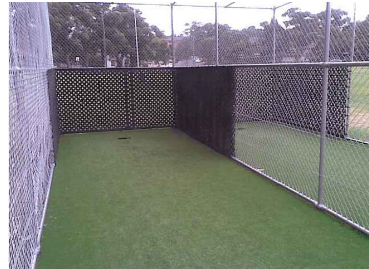
TYPICAL RUBBER BELTING - TO BE INSTALLED ALONG THE BATSMEN END AND EXTENDED 6.0m ALONG THE SIDES.
